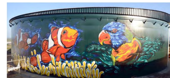
Bottom City Reservoir is a landmark, a public artwork and a functional reservoir overlooking Townsville, Queensland
