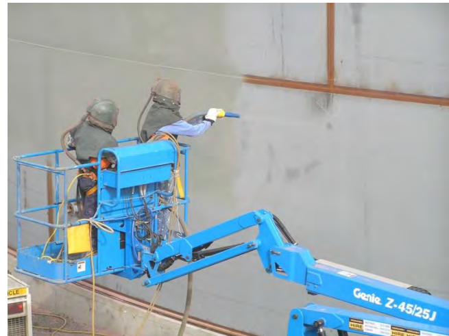
Spot abrasive blast cleaning on Mount Ridley Potable Water Tank Vic
