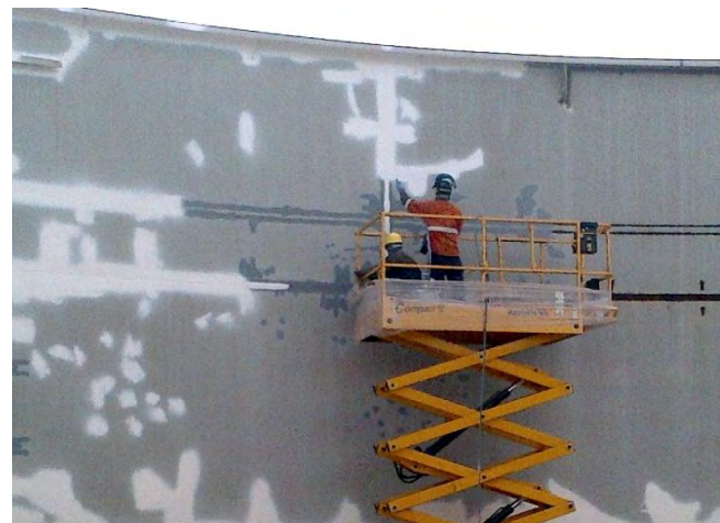
Spot abrasive blast cleaning on Werribee Water Tank Vic
