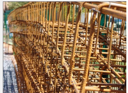
Concrete buildings contain almost as much steel as steel buildings
