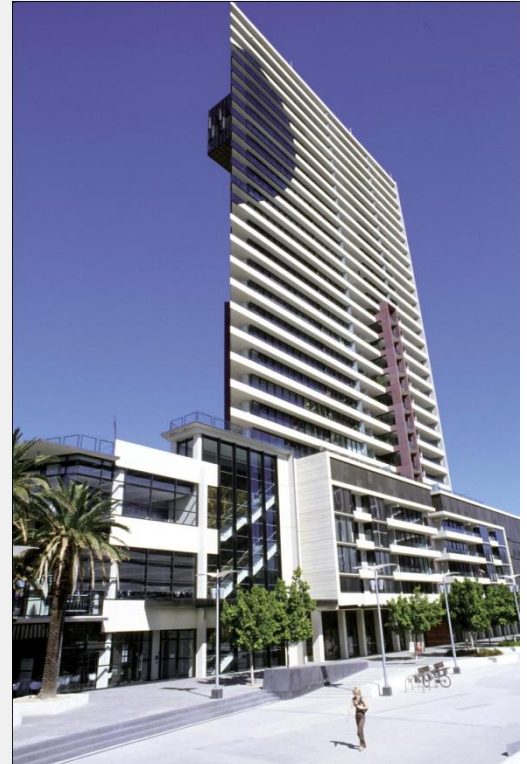
Yarra's Edge steelwork is protected against corrosion with both galvanic protection using a zinc rich primer and barrier protection using a high performance epoxy.
