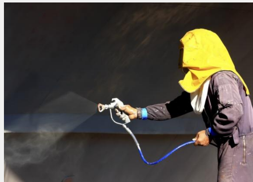
Wearing the correct personal protection equipment according to State laws will prevent inhalation of atomised paint particles and solvent
