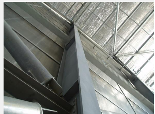
The eco designed Tallawarra Power Station's steelwork – Aquagalv.
