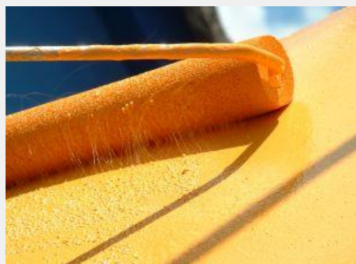
If the paint dries out too quickly during application, it becomes too thick and stringy to allow a good finish
