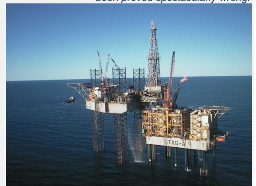
Off shore platforms are often protected against corrosion by high build glass flake epoxy, which offers outstanding barrier protection. Sacrificial methods are inadequate in such an environment.
